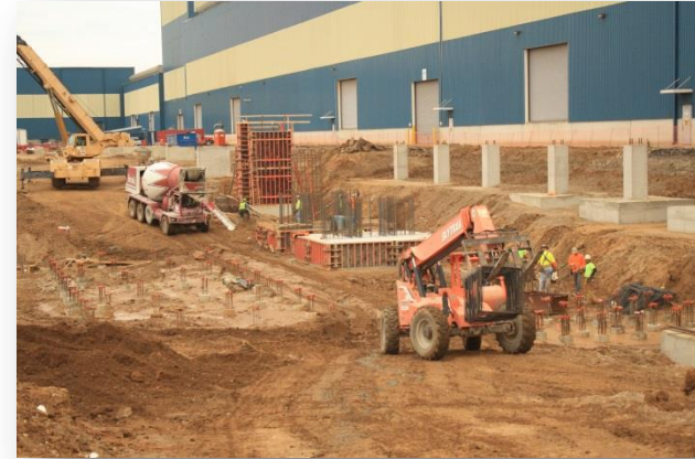
ZM construction, NAS
