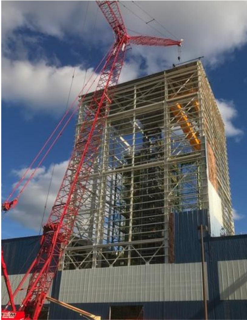
BA construction, NAS
