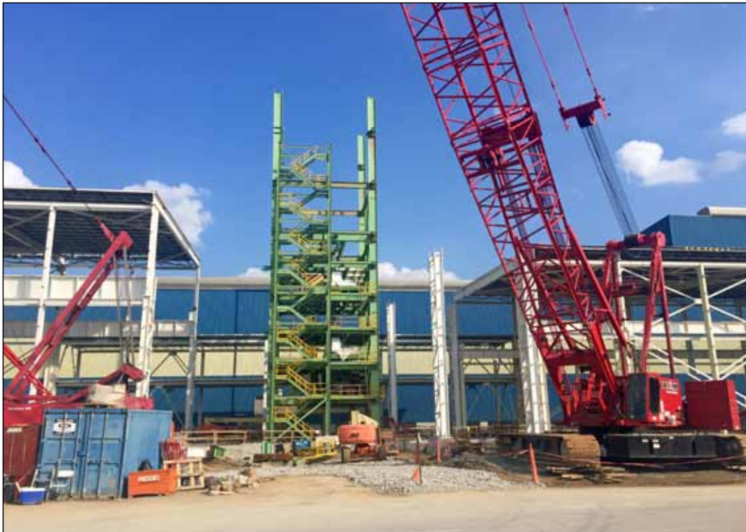
NAS Factory, construction of furnace in BA line.
