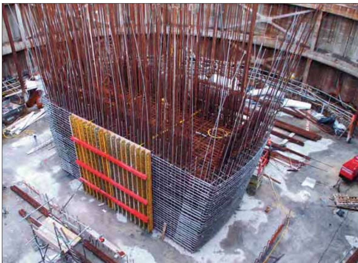
Corrugated stainless steel wire rod used for reinforcing the structure of the "Queensferry Crossing" bridge (Scotland).
