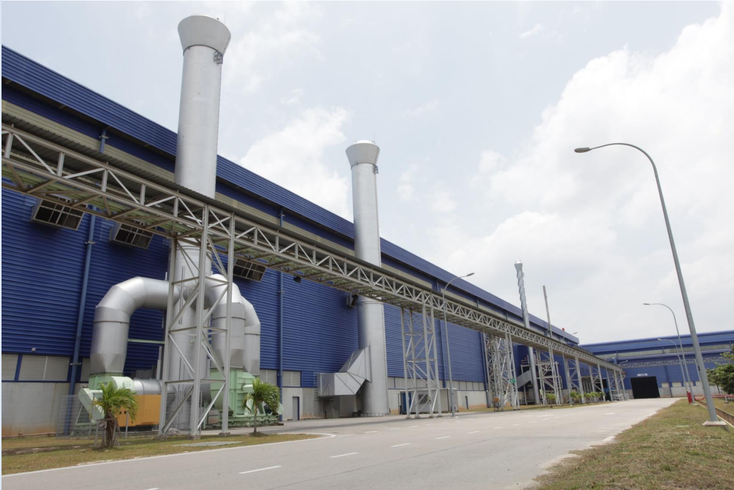
Stainless steel chimneys at the Bahru Stainless factory
