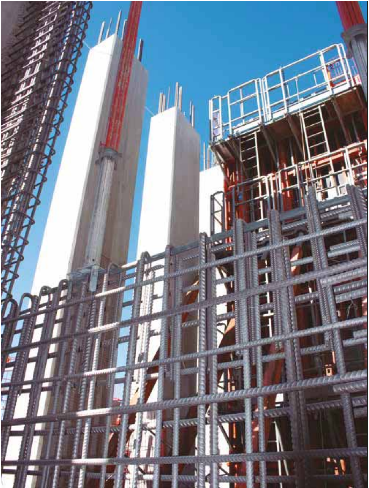
Stainless steel reinforcing bars from Roldan for the extension of Anse de Portier in Monaco.
