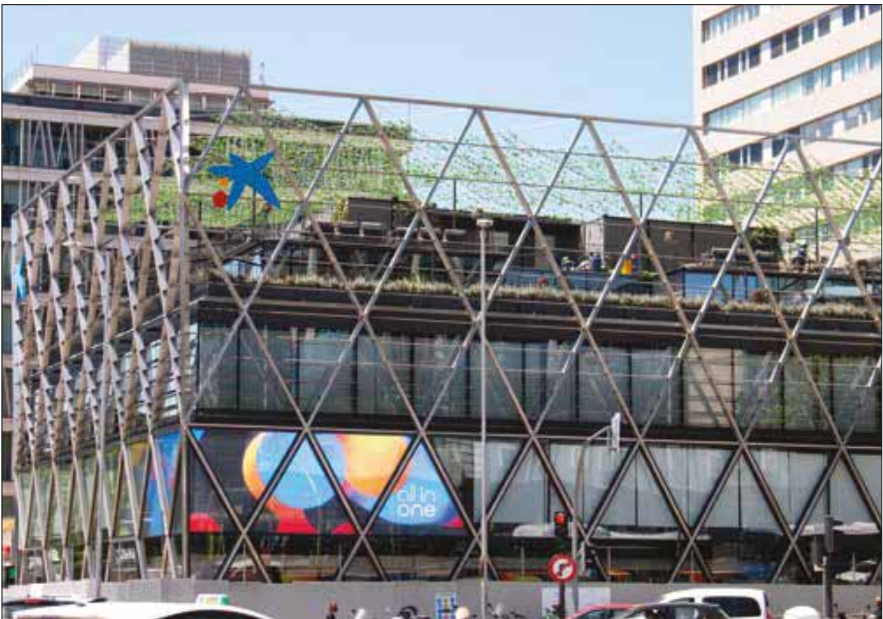
Stainless steel façade produced by Acerinox for Plaza de Colón in Madrid (Spain).
