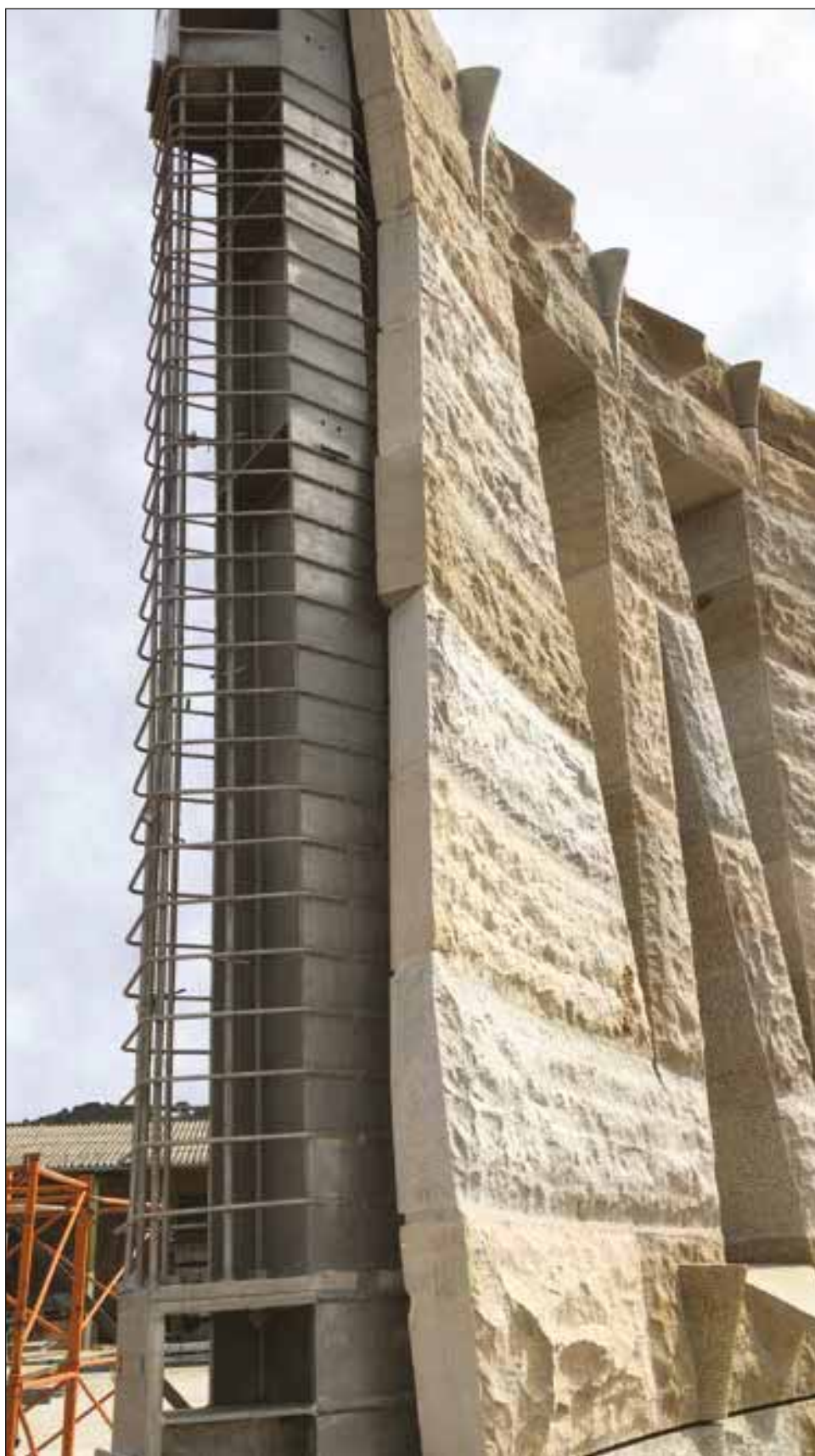
Reinforcing ribbed bars from Roldan as Stainless Steel reinforcements used in the construction of the Sagrada Familia Basilica in Barcelona (Spain).
