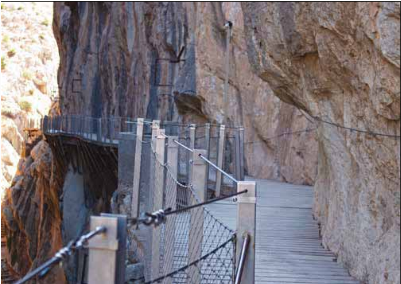
Railing made from Stainless Steel Flat Bars and Stranded Wire at the "King's Path" in Málaga (Spain)
