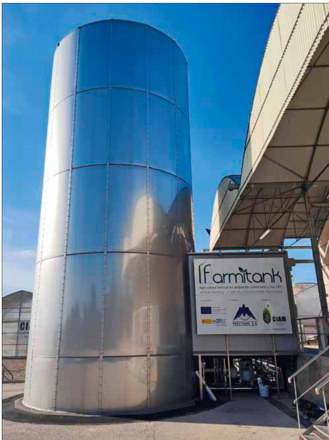
Tank for vertical Agriculture made of Stainless Steel produced by Acerinox Europa.
