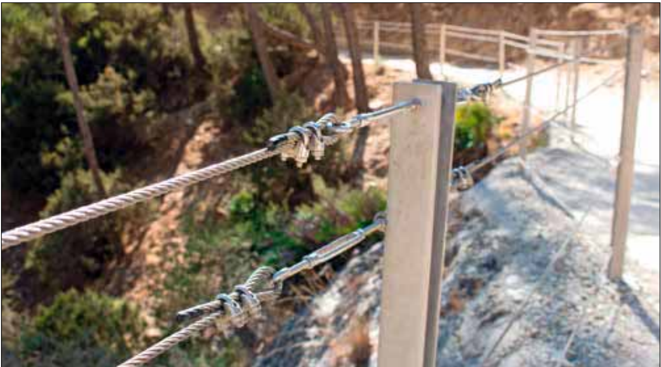
Railing made from Stainless Steel Flat Bars and Stranded Wire at the "King's Path" in Malaga (Spain)
