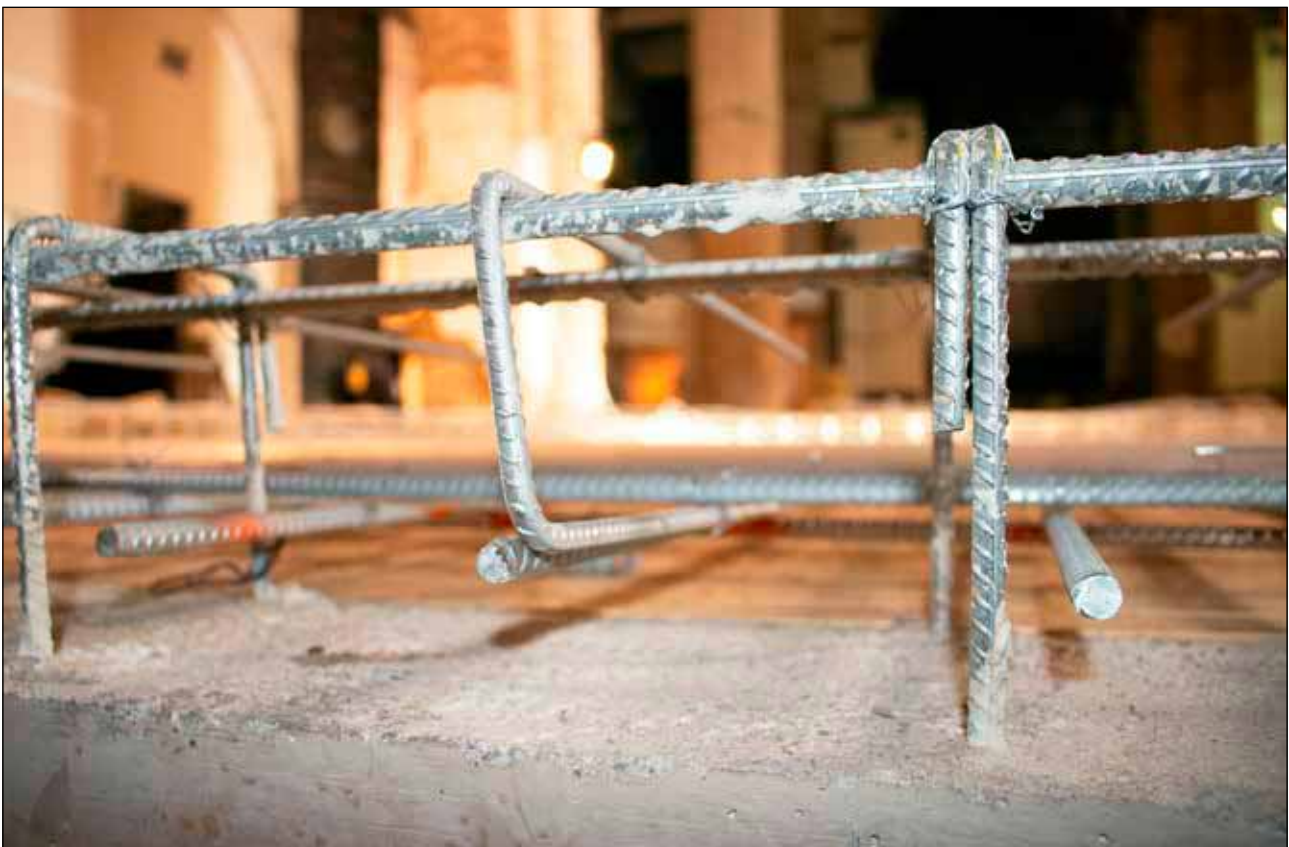
Corrugated Stainless Steel made by Roldan, used for the restoration of the Church Santa Catalina in Seville, Spain.
