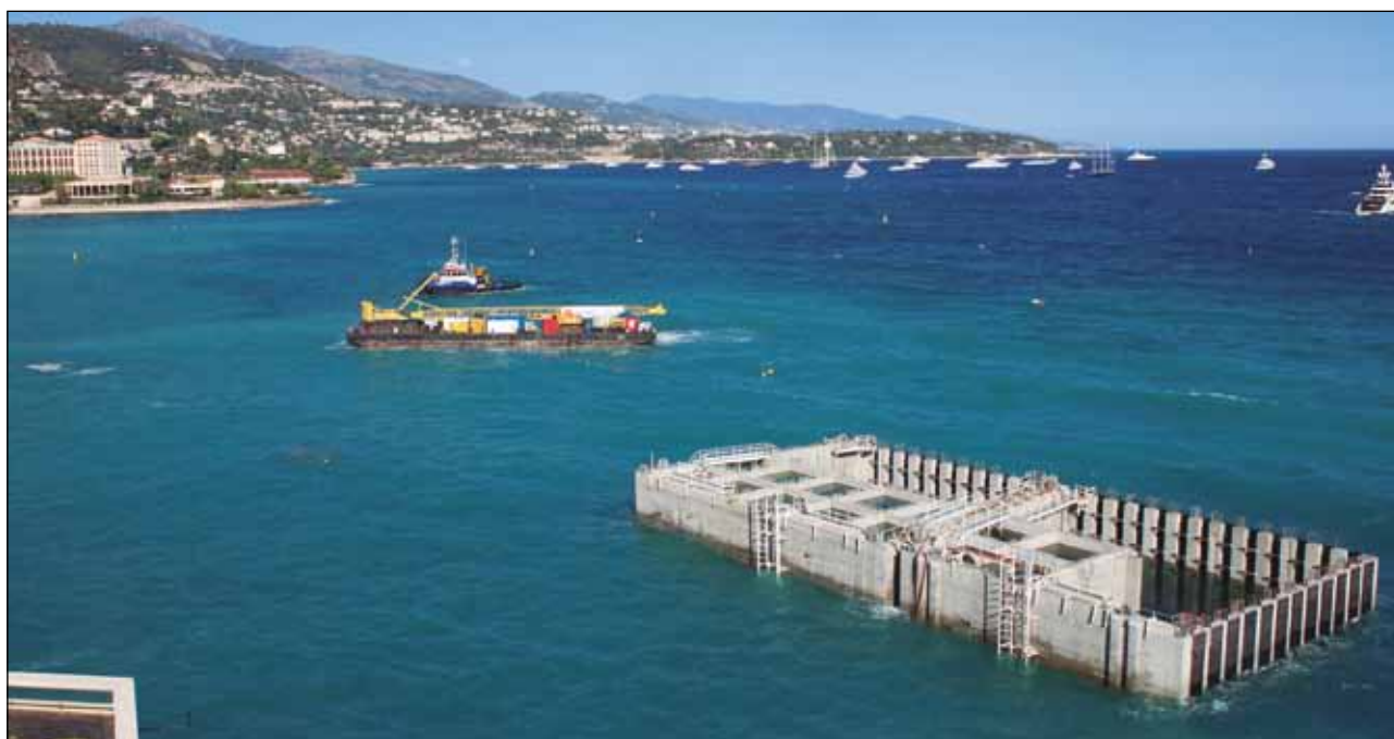
Reinforced Concrete Crate with reinforcement of stainless Steel reinforced bar for the Monaco Harbour
